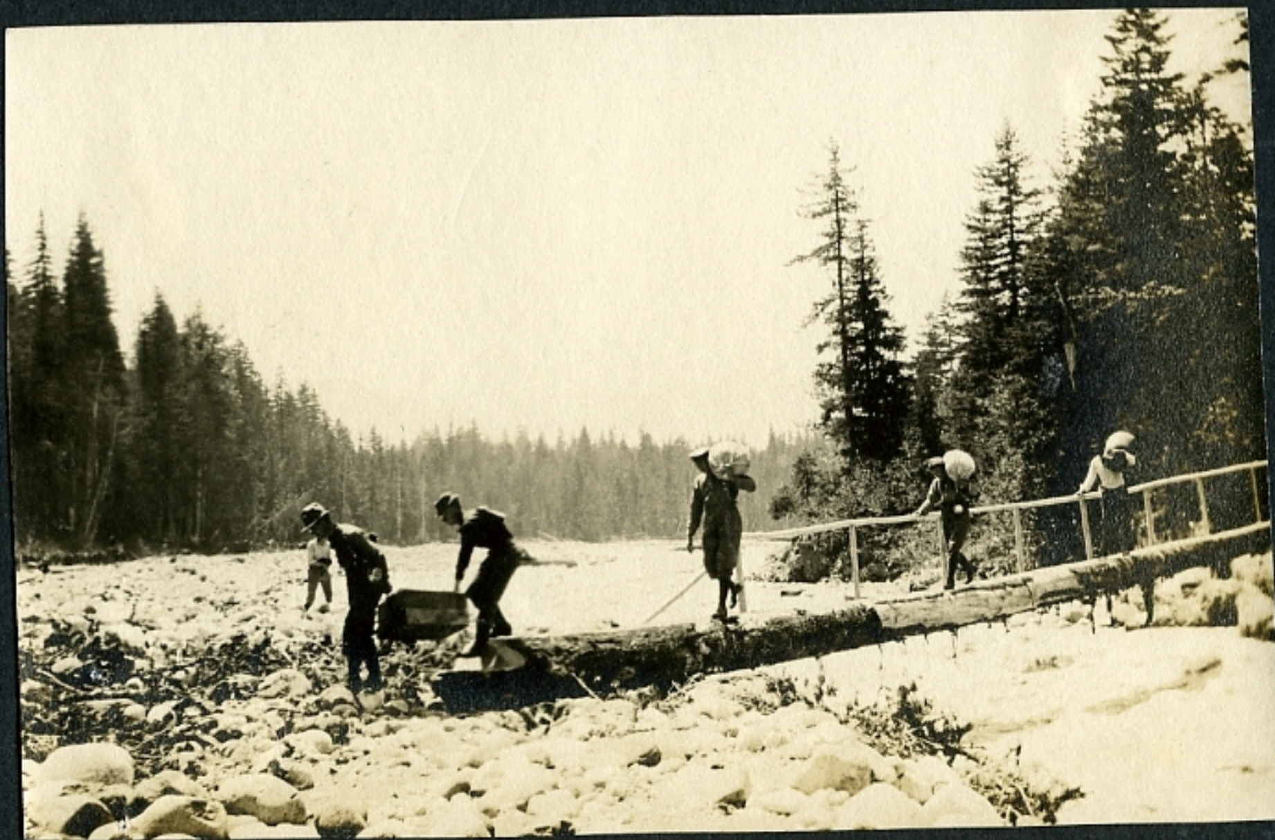
Carrying dunnage across the Nisqually River
