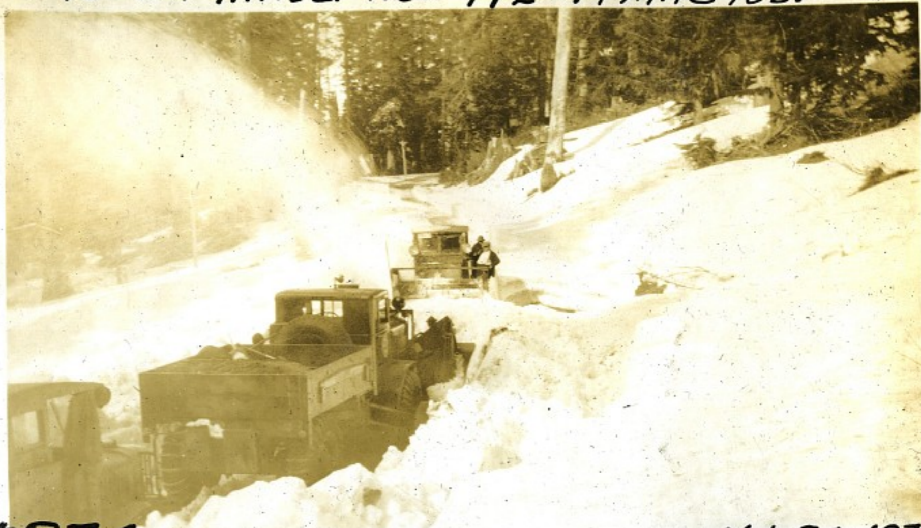
S.R.#15 - In Timber near Tye - 14 Mile Post
