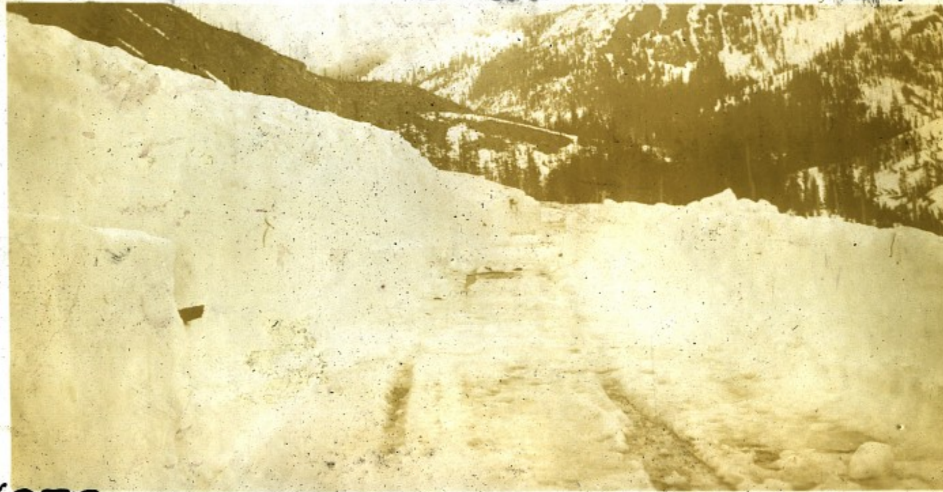
S.R. #15 - Stevens Pass, near site of old Crusher Plant
